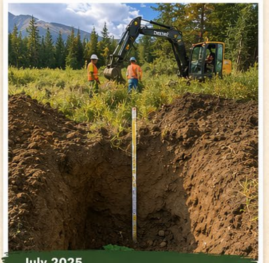
July 2025 Test Pit work to inform septic field design
